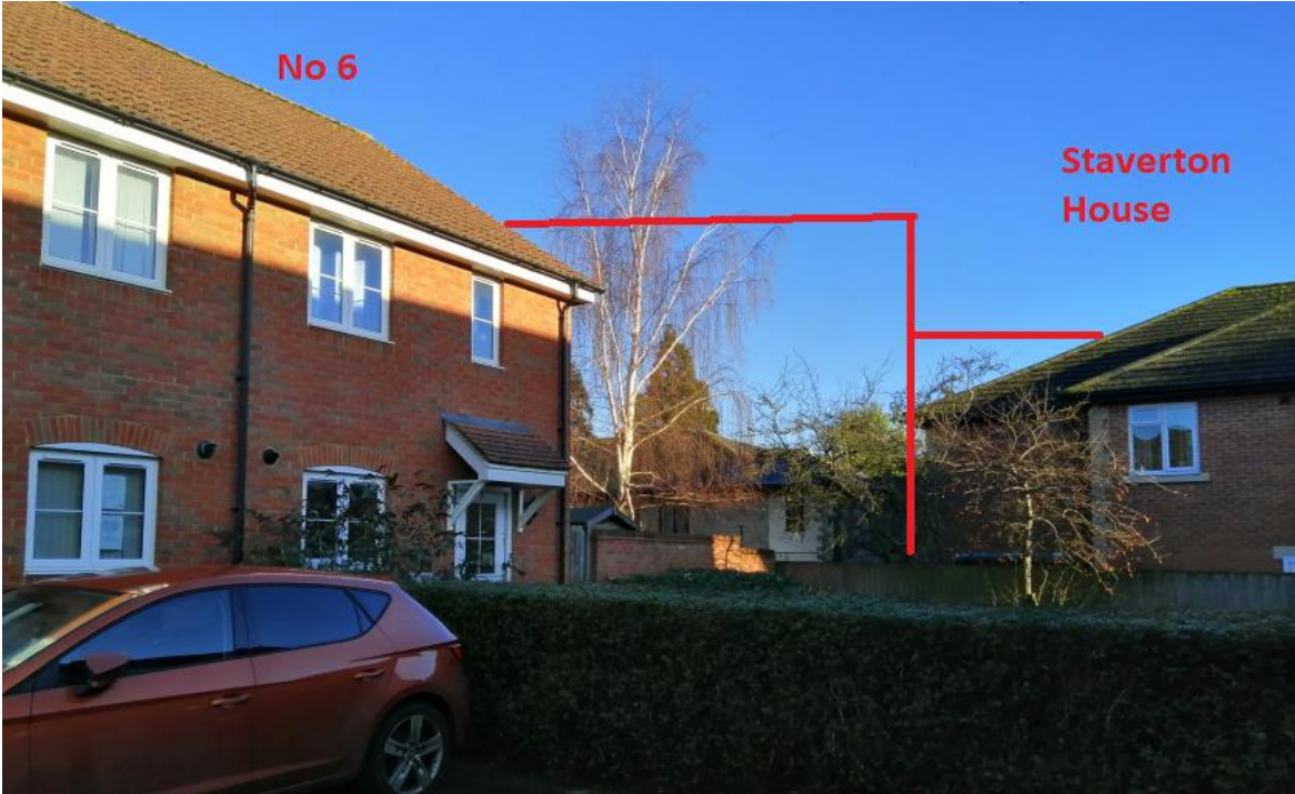
Photo of No 6 (left), Staverton House (right), existing single storey section (centre) with Officer drawn approximate outline of proposed 3 storey central section
